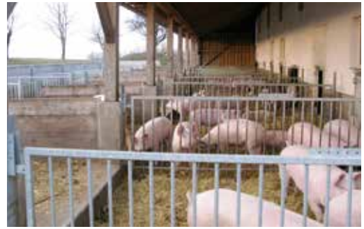
Example of a fattener pen with a covered outrun. Each unit has an exit to a separate outdoor run. In this example, the lying area is indoors.
